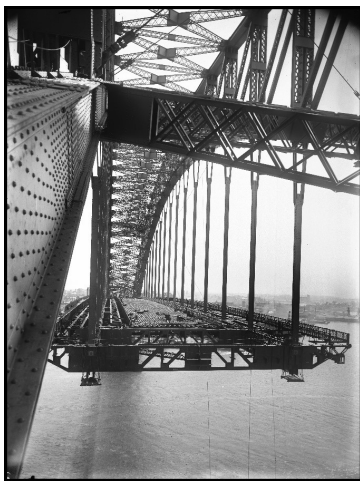
Sydney Harbour Bridge – decking from a cross lateral, Thursday 11 th Dec 1930. Photography by Rev. Frank Cash
