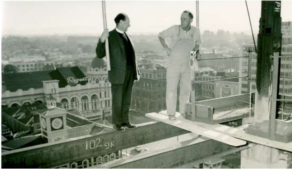
Rev K A Hadfield standing on a steel girder overlooking Cathedral Square, Christchurch, during the construction of the Bank of New Zealand building, 1966 [PCANZ Archives, P-A120.25-51]
