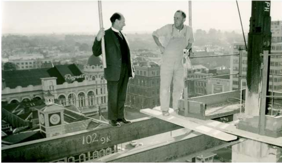
Rev K A Hadfield standing on a steel girder overlooking Cathedral Square, Christchurch, during the construction of the Bank of New Zealand building, 1966 [PCANZ Archives, P-A120.25-51]
